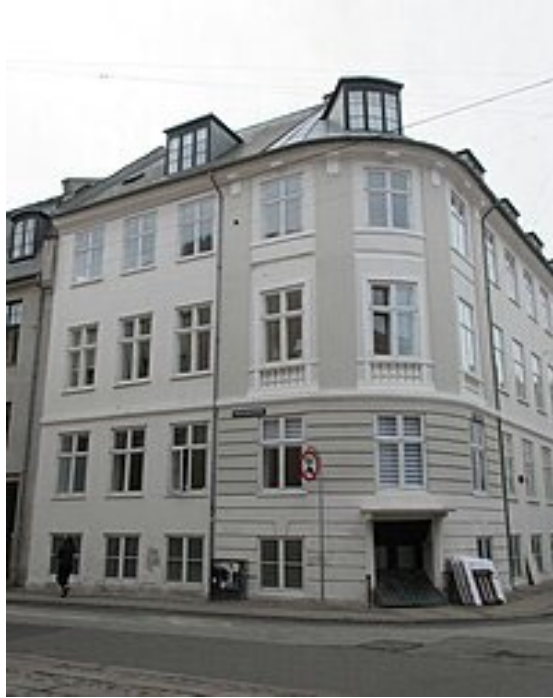
Lavendelstræde 1, Copenhagen, on the corner of Hestemøllestræde, where Constanze and Georg Nissen resided in the 1 st floor corner apartment
